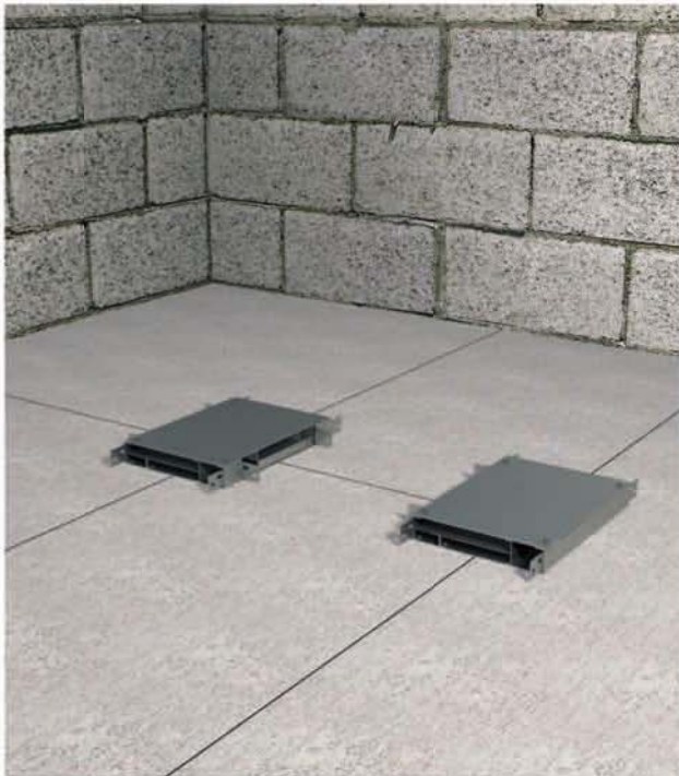
Step 2: Mounting of underfloor boxes
